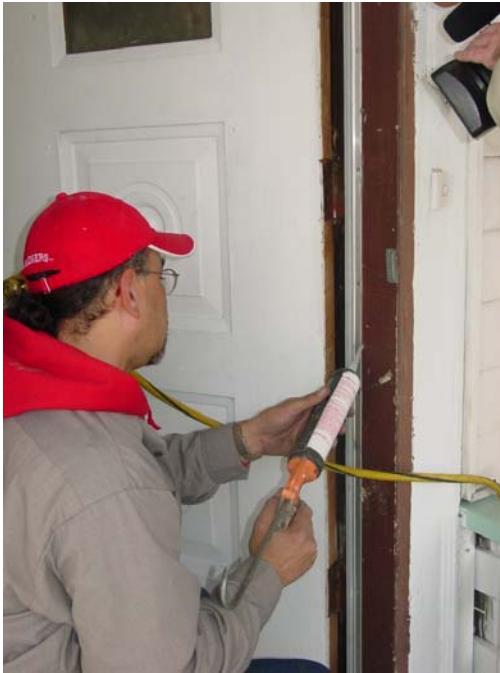
Resident applies caulk to improve weather-stripping of a home's exterior door.
