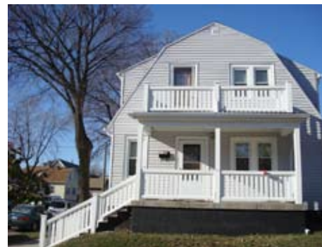
Southside home before and after work by NIP program.
